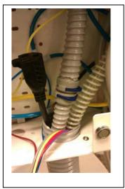
17. Remove the cap from the large water supply line, Connect the water supply line to the cuspidor. Remove the cap from the signal air line, then connect it to the cuspidor.
