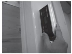
Fig. 3 -31: Checking for column lean (front)
