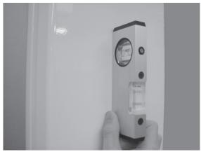
Fig. 3 -26: Checking for column lean
