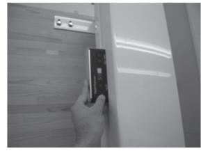
Fig. 3 -30: Checking for column lean (sides)
